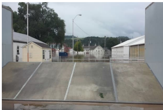
Figure 4-4: Flip Up Gates, Bloomsburg, Pennsylvania, FloodBreak
